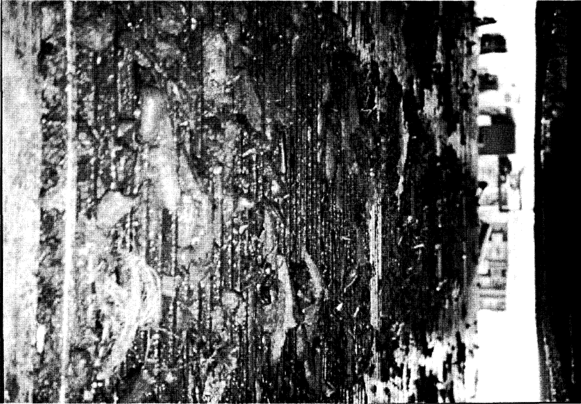
Photo 4. Debris Clogged Fish Unit Trash Rack
