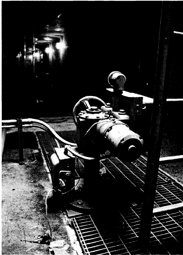
H5 Diffuser B Gate Actuator
