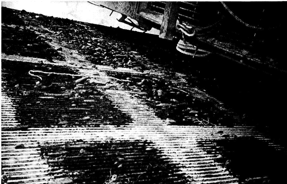
H3 Plugged Traskrack
